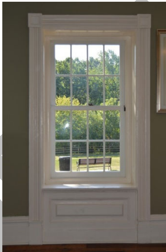
Photograph 17. A detailed view of a window in the west parlor (Room 103), looking southeast.
