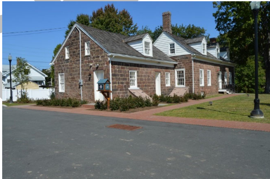
Photograph 6. Oblique view of the side (southeast) and front (southeast) elevations of the Garritse/Doremus/Westervelt House, looking north.
