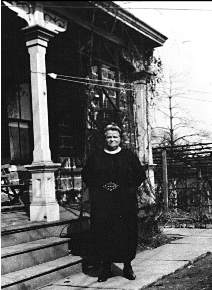
Figure 4. Maria Martin standing outside of the Garritse/Doremus/Westervelt House near one of the Italianate-style porches. Circa 1914-1930. Source: New Jersey Historic Preservation Office 2019.
