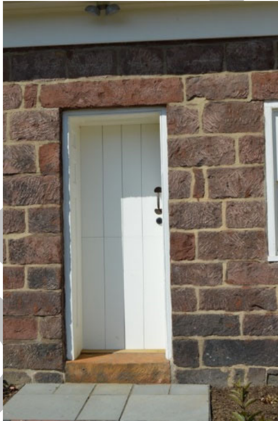
Photograph 9. The non-original Dutch door on the front (southeast) elevation of the kitchen wing, looking northwest.
