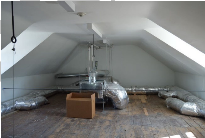
Photograph 11. The kitchen wing garret, looking northeast.
