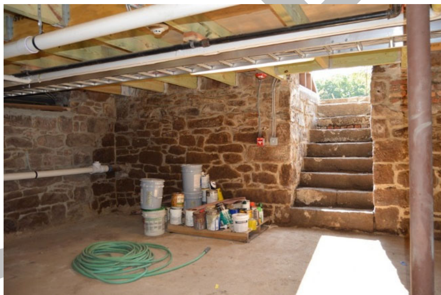
Photograph 22. The kitchen wing basement (Room 003), looking east.
