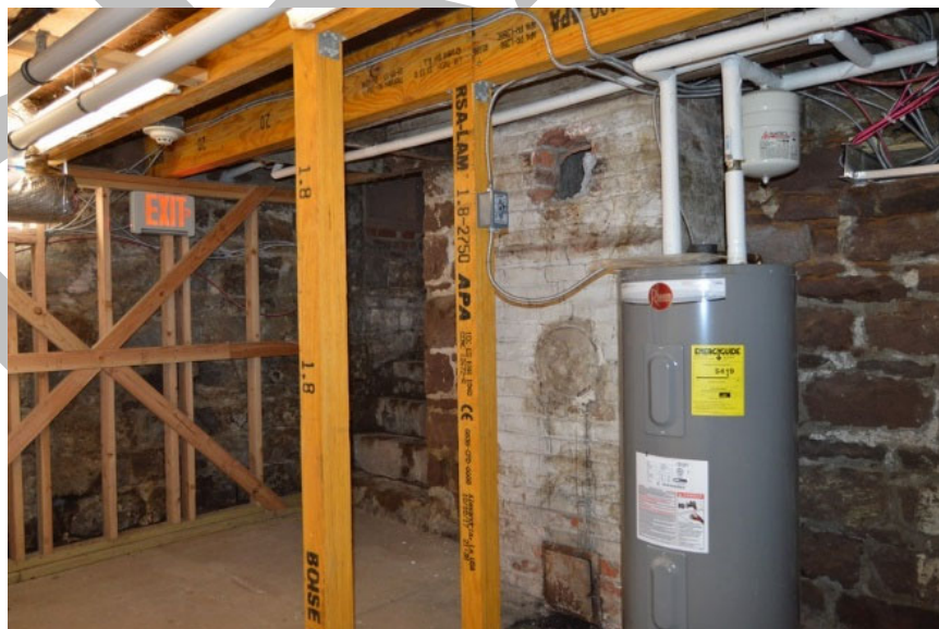
Photograph 21. The basement of the building's main block (Room 002), looking south.
