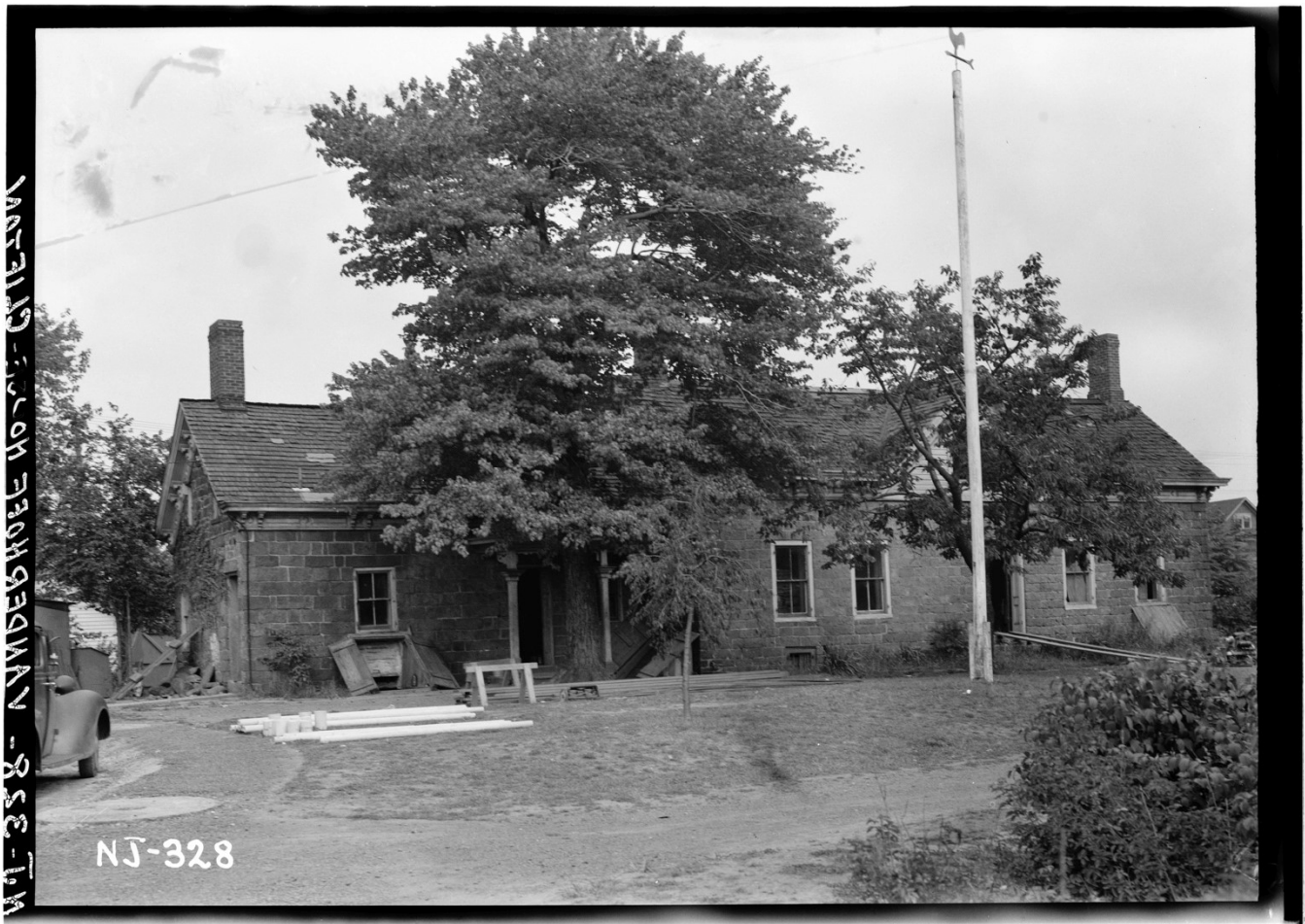
Figure 6. The front (southeast) elevation of the Garritse/Doremus/Westervelt House. August 18, 1939. Source: Historic American Buildings Survey.
