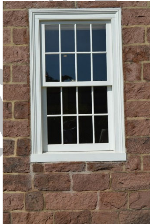
Photograph 8. The window to the left of the primary front entry, looking northwest.
