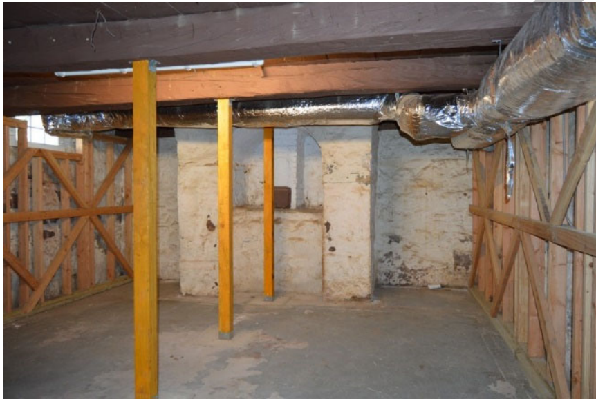
Photograph 20. The basement of the building's main block (Room 001), looking northeast.
